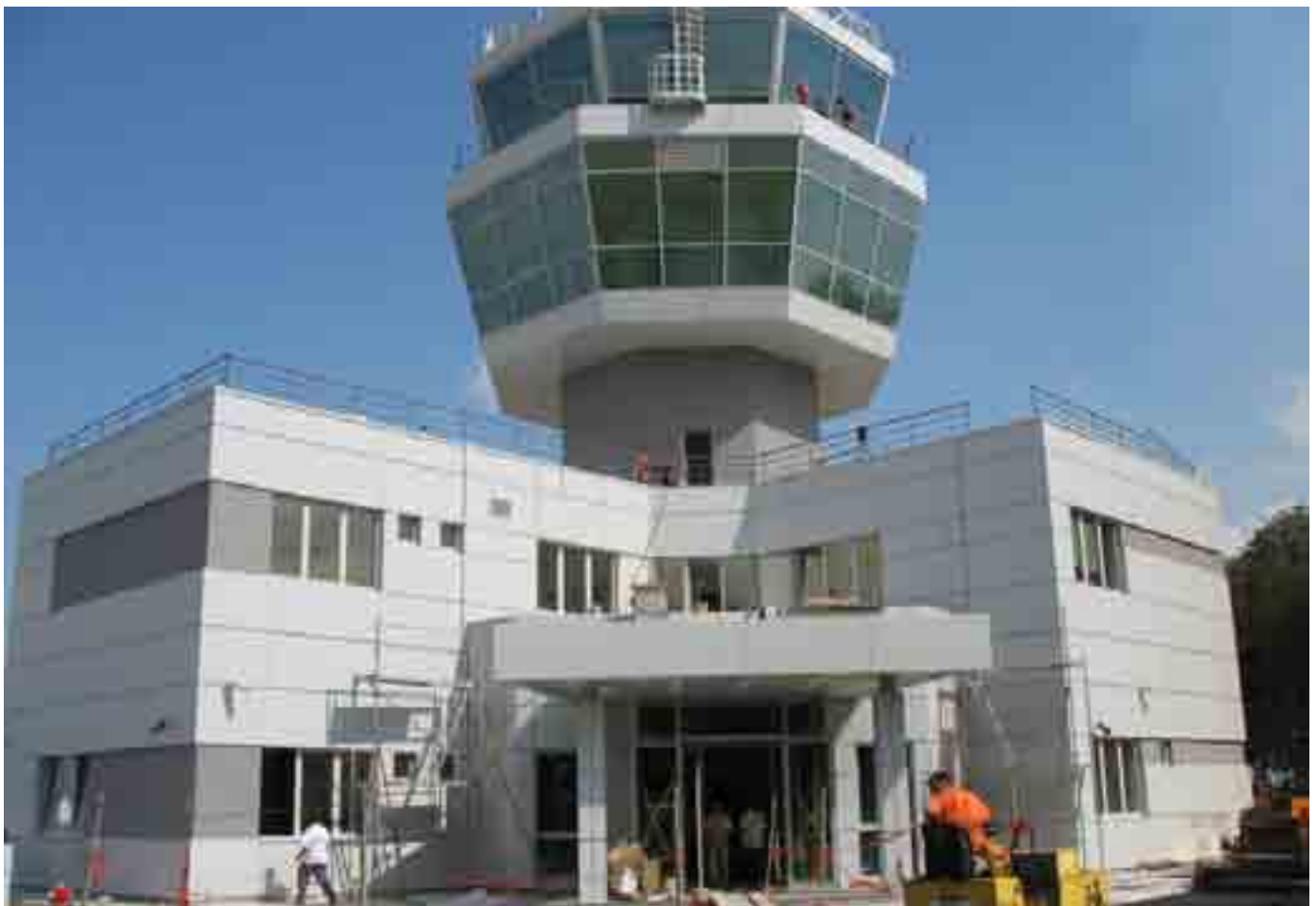
Figure 27. New TWR Construction at Airport Batajnica
